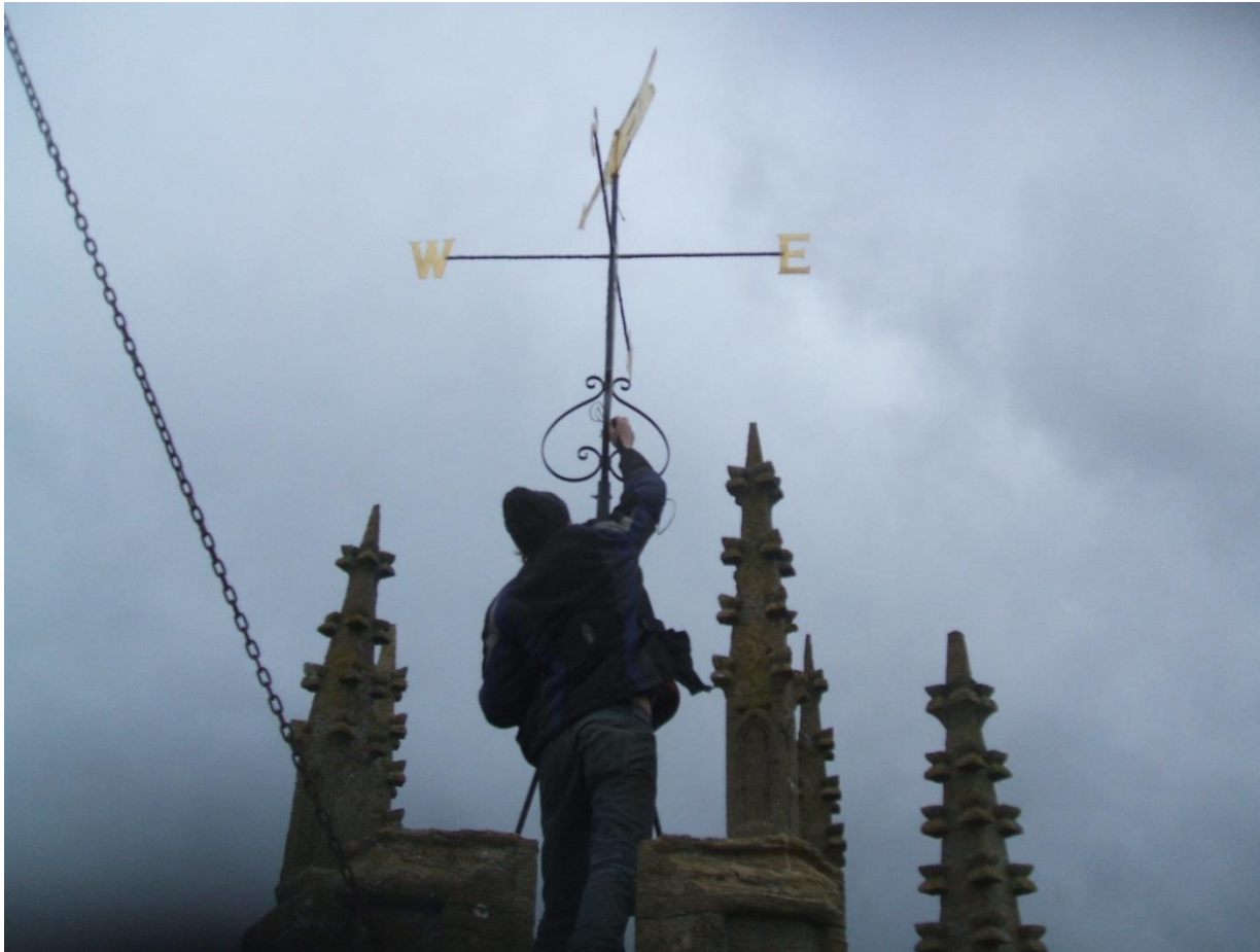
Weather vane repair and refurbishment
